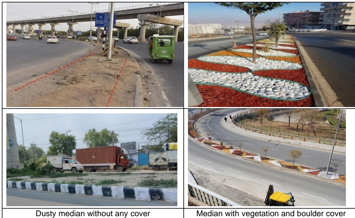
Plate 5.3: Median condition after boulder dressing
